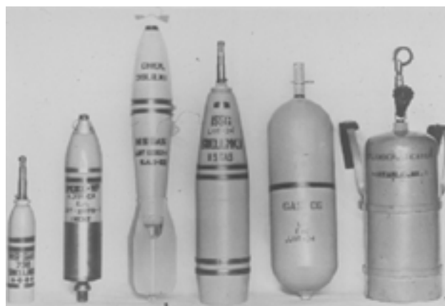
Fig. 2-18. The chemical weapons of the 1920s and 1930s. From left to right: the 75-mm mustard shell; the 4.2-in. white phosphorus shell; the M1 30-lb mustard bomb; the Mk II 155-mm mustard shell; the Livens phosgene projectile; and the Mk I portable chemical cylinder. Photograph: Chemical and Biological Defense Command Historical Research and Response Team, Aberdeen Proving Ground, Md.
